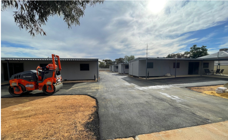
Asphalting of the driveway at Yalambee Units.
