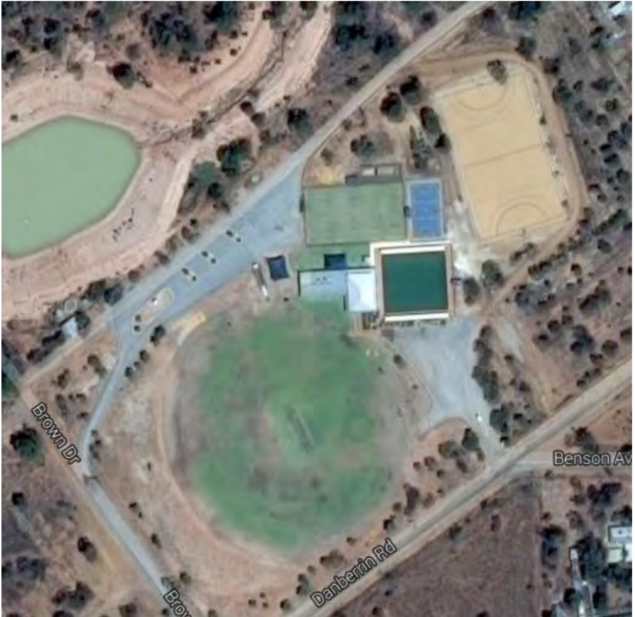
Photo 4: Aerial view of the Nungarin Recreation Complex
