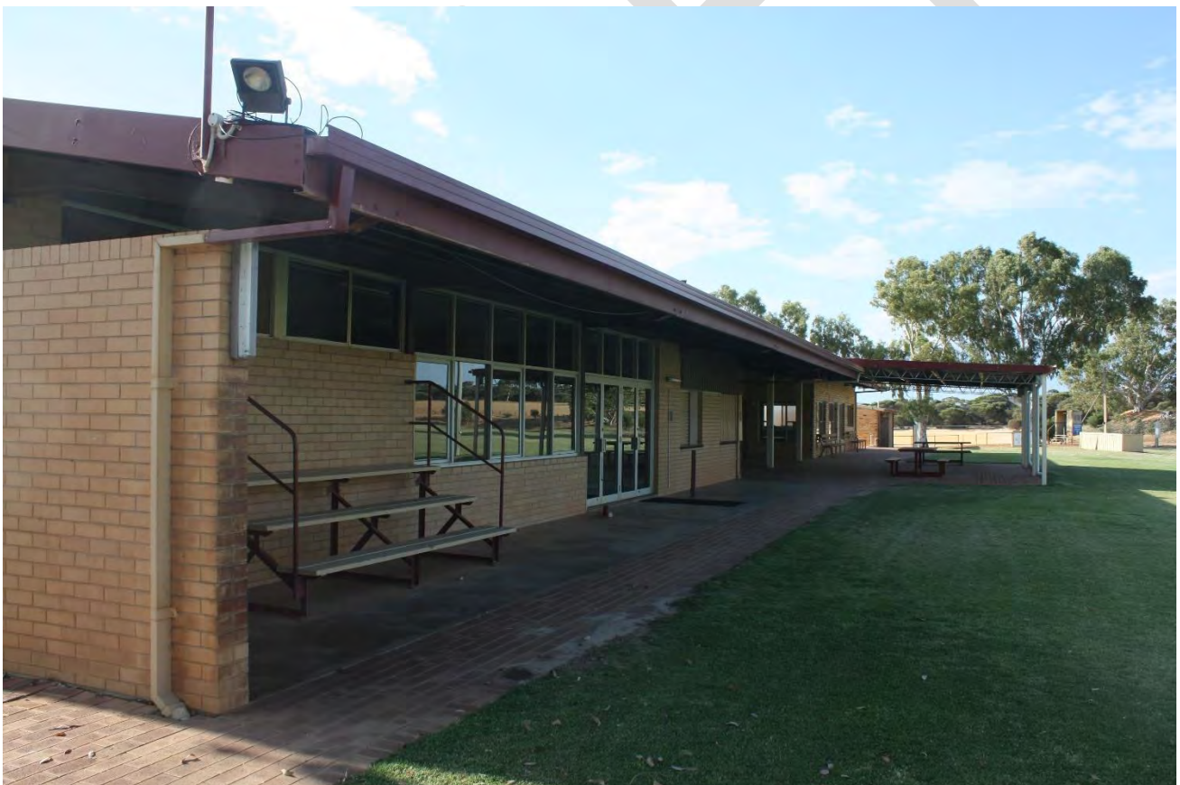
Photo 1: Existing sports clubroom facility
