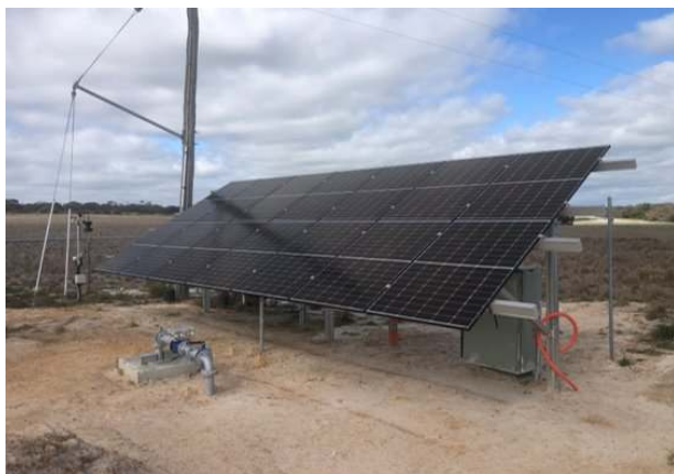
Parker Road Bore
